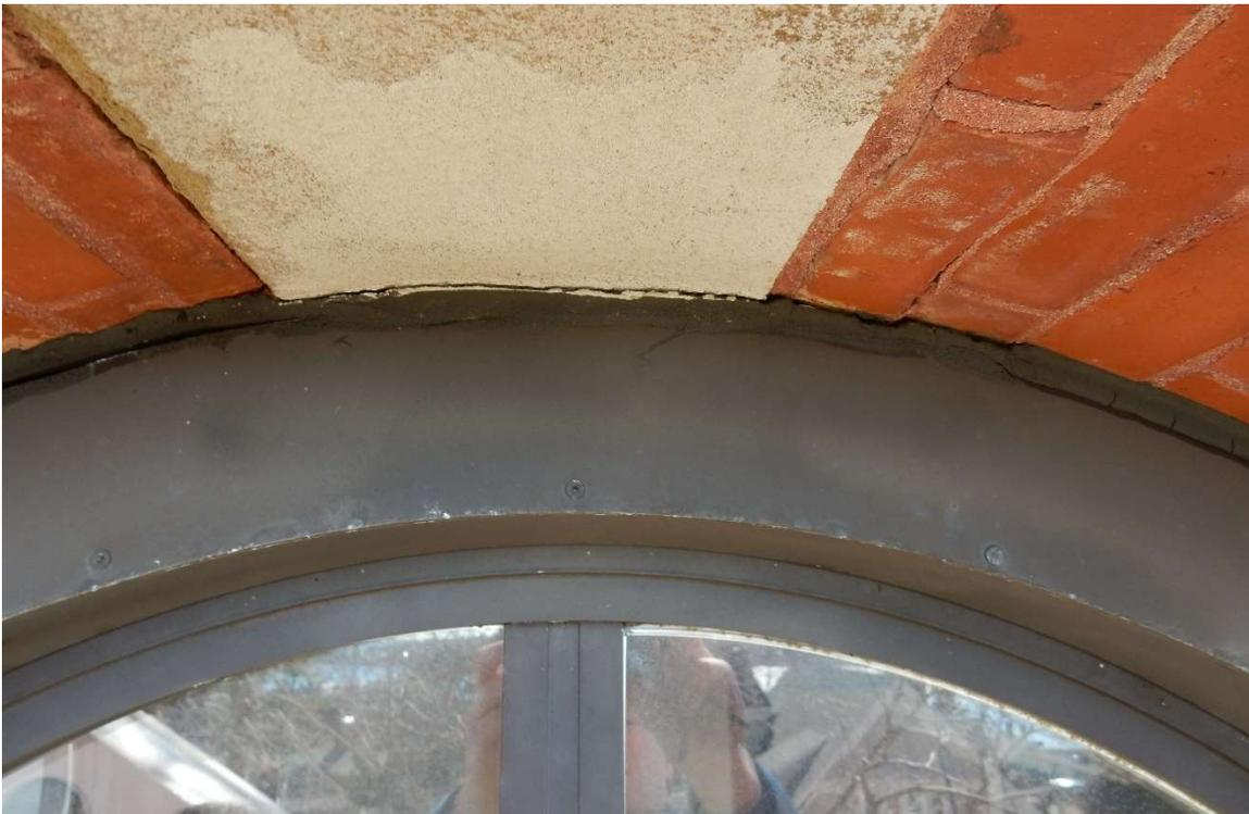
Failed Sealant at Perimeter of Windows
