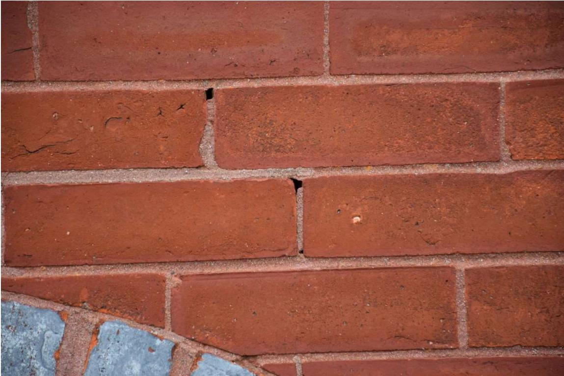
Failed Mortar with Hollow Backup
