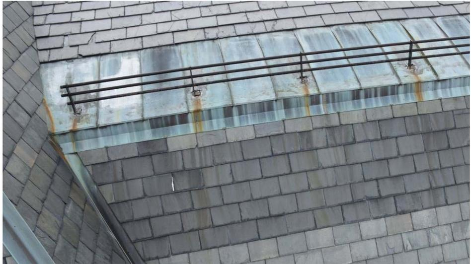
*Low Sloped Roof Deteriorated Skirt and Snow Guard*
