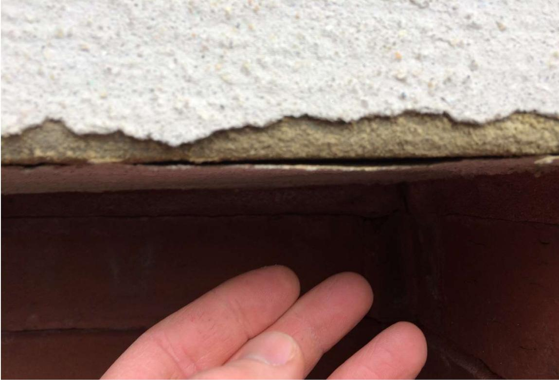
Delamination of Stone Caused by Coating
