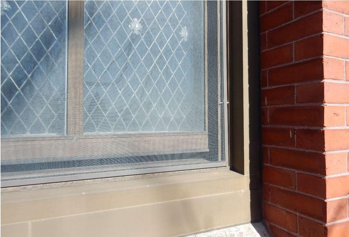
Seal Failure at Window Glass and Window not
