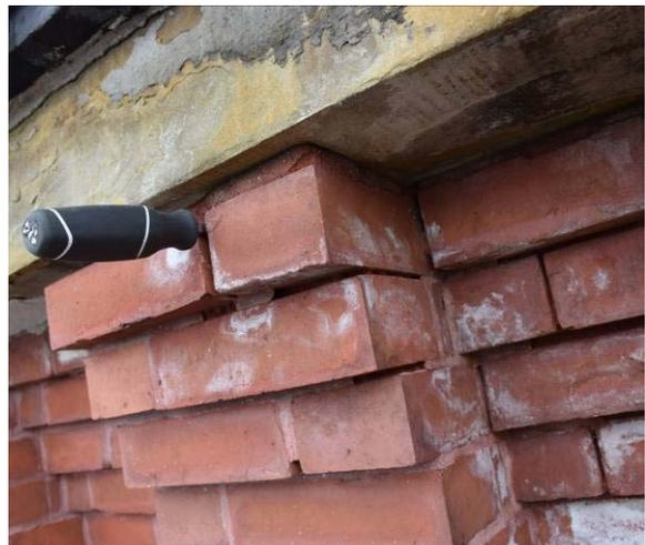
*Open Cornice Joints at Corbel with Loose Brick*
