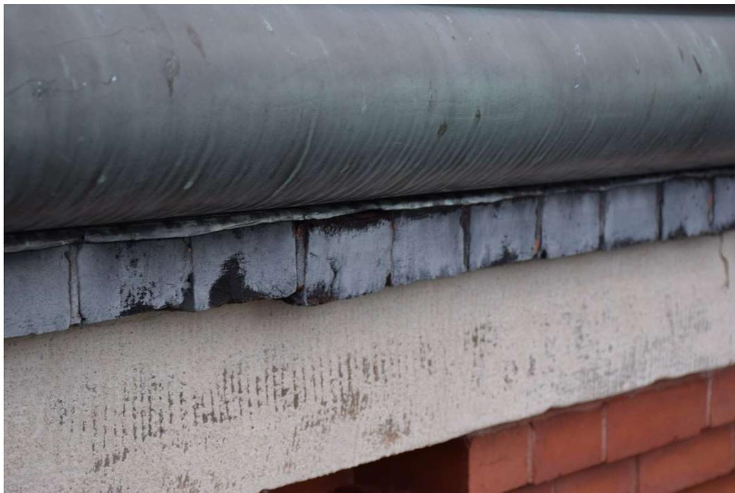
Movement of Brick Below Gutter
